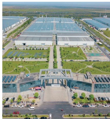
Haining phase four 3-5GW Biggest capacity in one house
